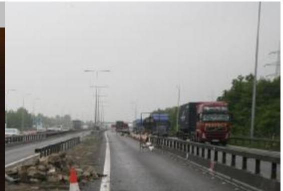
Progress picture (May 2010)
